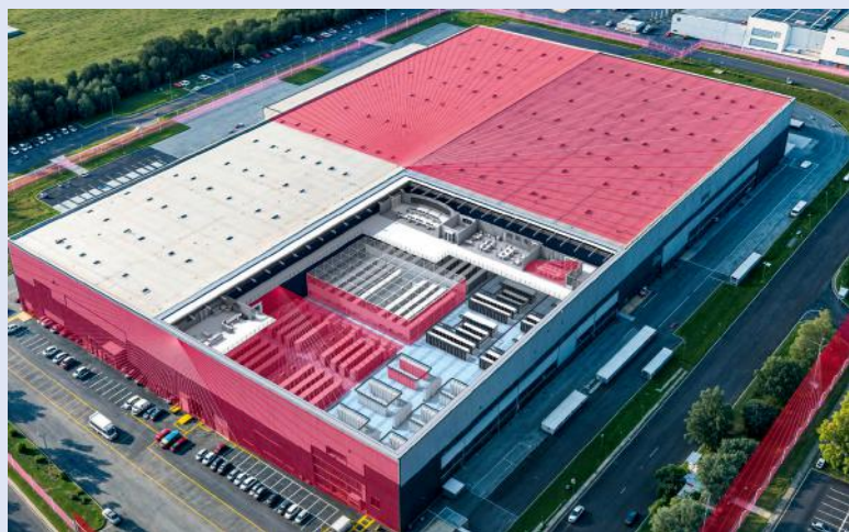
As datacentres expand into remote and rural areas, the need for adaptable and scalable security solutions continues to grow.
