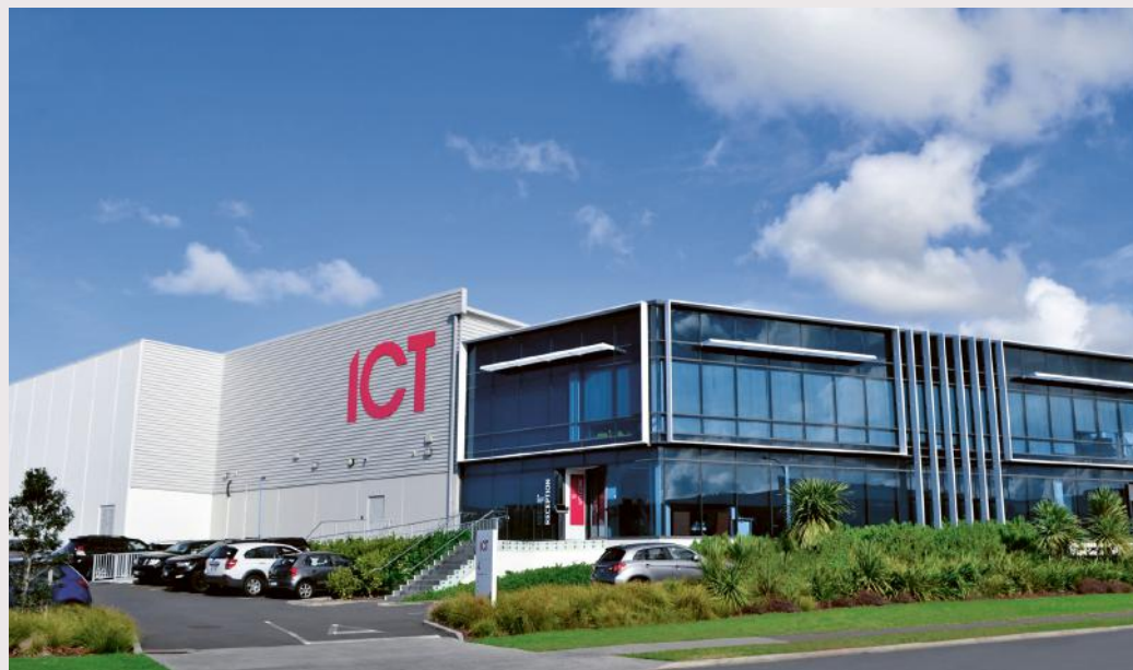
ICT's headquarters and manufacturing facility in Auckland.
