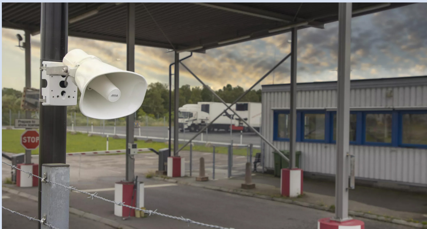
Network audio can be configured to trigger alerts that tell operators to visually assess a situation and then speak directly to the individuals involved via the speakers.
